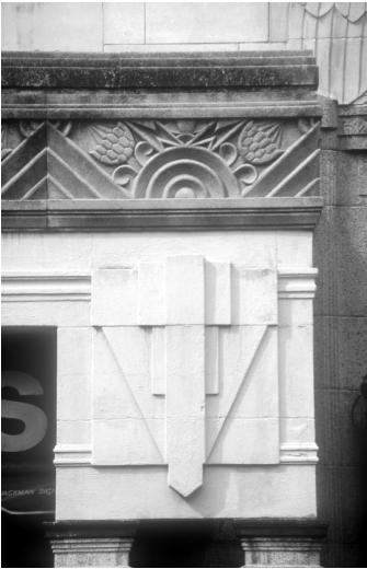
Figure 13 Grant, Commercial Union Building, detail of façade moldings, 1932
