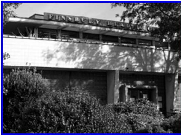
Figure 10 Finsbury Health Centre, front. Photograph © James Mosley, 2005.
