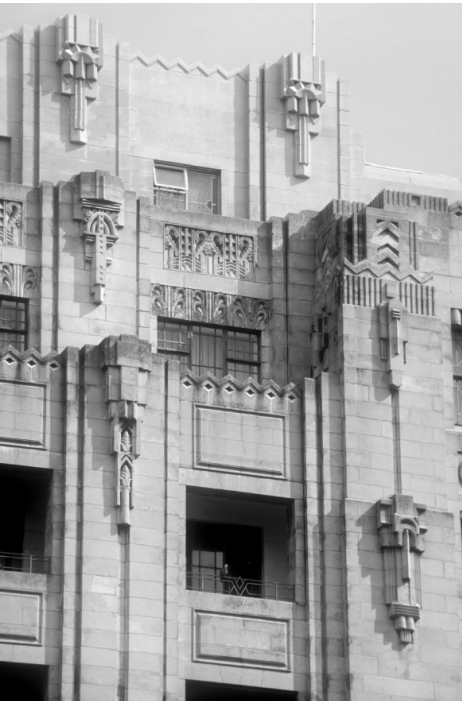
Figure 11 (above) Grant, Commercial Union Building, detail of stepped parapets, 1932
