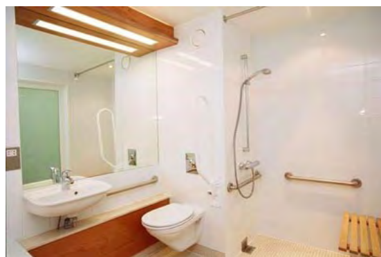
Figura 5: Sanitario accesible. Fuente: disponible en http://www.owensbuildingservices.co.uk/devon-disabled-kitchen-bathroom/devon-disabled-bathrooms.html
