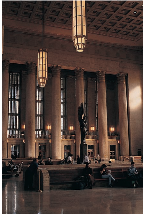
Plate 9. The renovated luminaires in this Philadelphia railway station are switched on all day, even though the daylight streaming in through the windows provides perfectly adequate illumination
