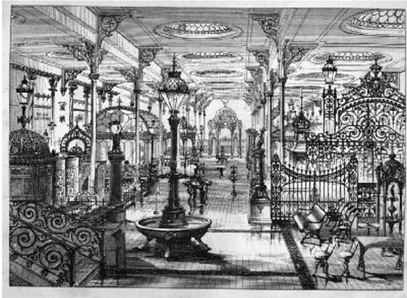
Figure 135 Walter Macfarlane and Co's premises, 1882.
