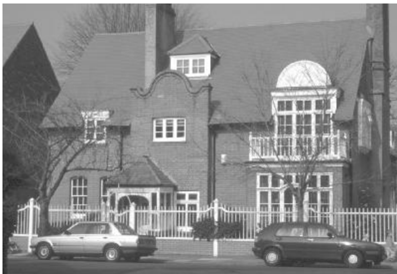
Figure 88 House in Bedford Park. (Courtesy of David Long.)
