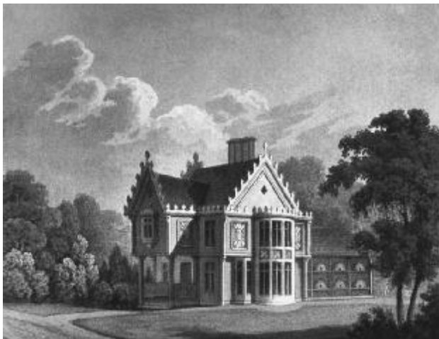
Figure 33 Small dwelling for William Currie, near Guildford, designed by Robert Lugar. (Courtesy of Cyfarthfa Castle Museum and Art Gallery.)
