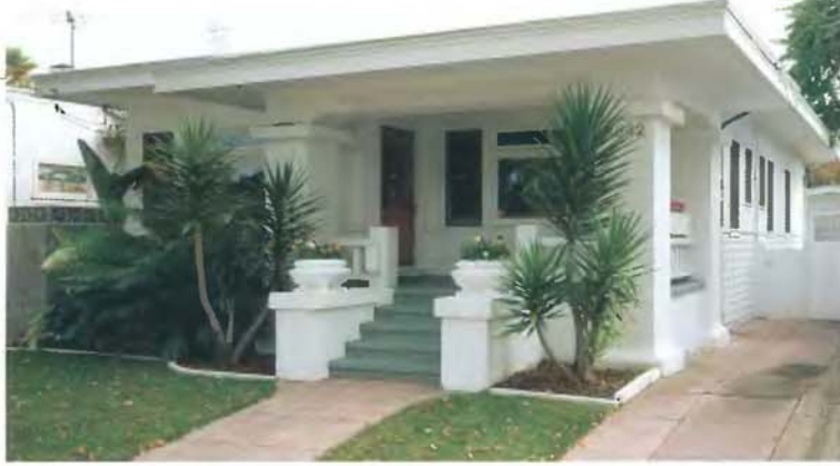
▲ This small Prairie Bungalow is all roof and columns, with its exaggerated overhang and strong front-porch pillars. Oversized planters frame the steps leading up to the outdoor space, a typical Prairie touch.
