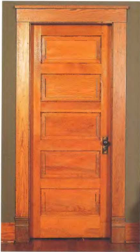
▲ The most common type of interior door in Bungalow-style homes has five evenly spaced horizontal raised panels inset into simple stiles and rails.
