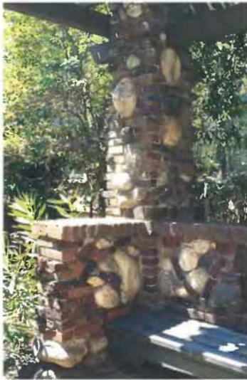
▲ A closer look at the porte cochere in this 1907 home reveals masonry work combining brick and river rock that was common to Southern California Bungalows.
