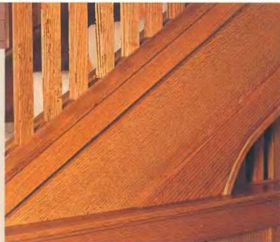
▲ A close-up view captures the fine grain of the quartersawn oak used in the construction of the staircase skirting.
