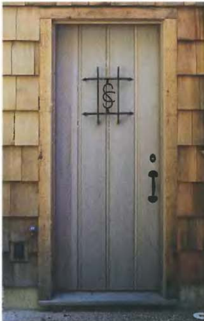
▲ A holdover from earlier styles, this simple batten door adorned with wrought-iron scrollwork and hardware provides textural contrast to the shingle siding, underlining the overall rustic look of the Arts and Crafts style. Photo © www.carolynbates.com , Sandra Vitzthum Architect, LLC.
