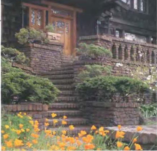
▲ Oak doors with colorful, geometric art-glass panes relieve the heavy texture of shingle siding and rough-cut stone used on retaining walls and walkways of this California Bungalow from 1912.
