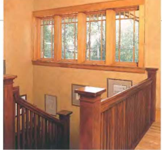
▲ Squared newel posts with oversized caps define each turn of this staircase.
