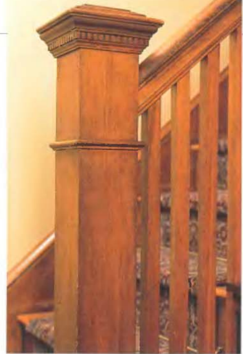
▲ The cap of the newel post in this 1915 Bungalow features a complex layering of moldings, giving it a distinctive profile with its pronounced cornice. Classically based dentil molding surrounds the base of the cap.
