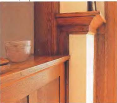
◀ The deep wainscot cap, which offers enough space to use as a display shelf in this newly constructed Craftsman-style home, is historically correct.
