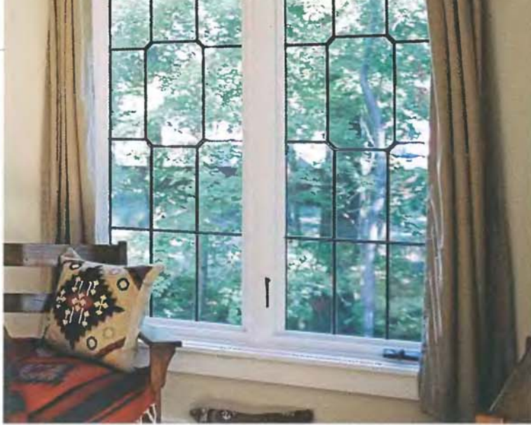
▲ Delicately shaped leaded-glass panes on these casement windows frame the view of the landscape, outlining each segment as if it were a fine painting. Photo © www.carolynbates.com , Sandra Vitzthum Architect, LLC.
