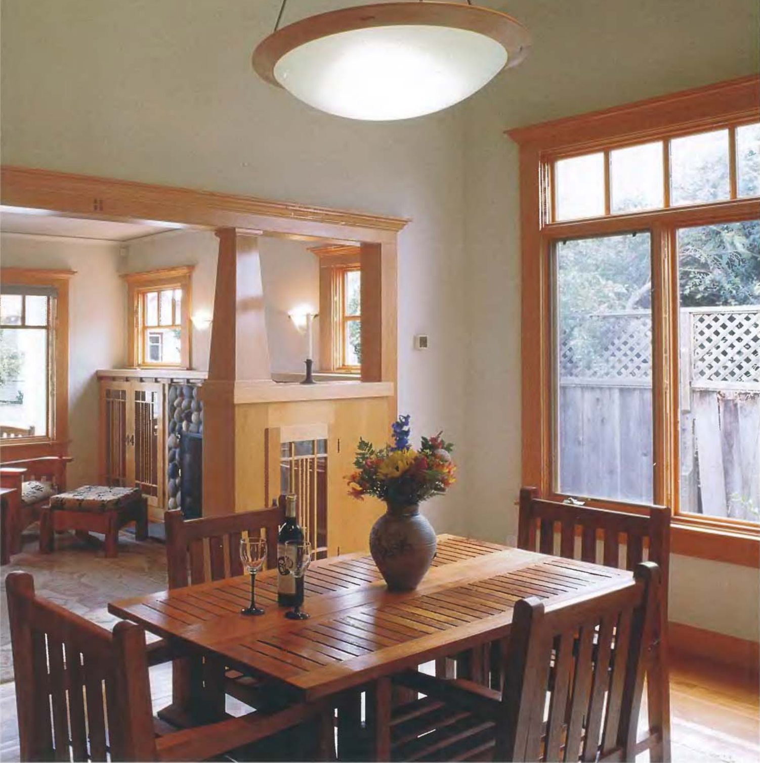
▲ Room dividers are designed to maintain a visual flow between spaces while offering separation between the dining and living rooms. The cased opening is capped with a deep cornice that matches the profiles of the window headers. Square, tapering columns lead the eye to glass-fronted built-ins below with Prairie style muntins.
