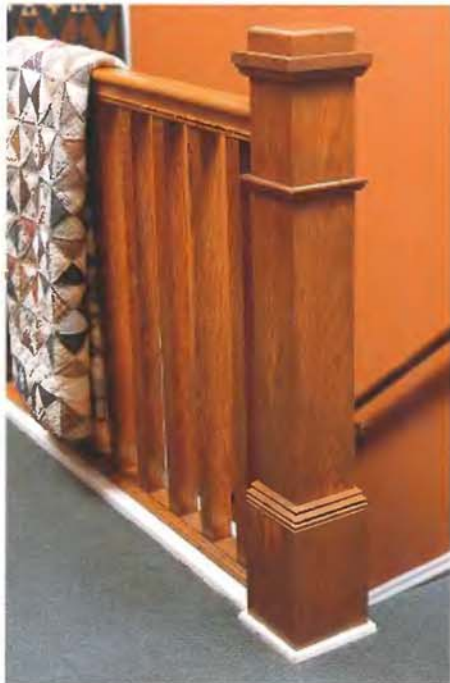
◀ A newel post on the upstairs landing is simple in its design compared with the one on the first-floor landing. ▼
