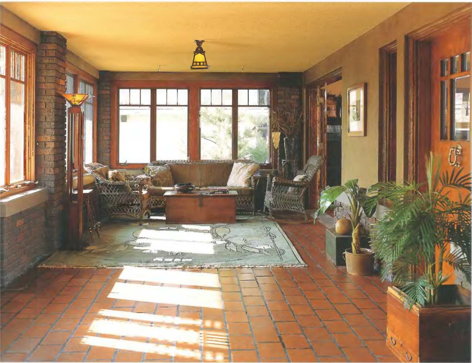
▲ Durable brick flooring in this entryway takes the brunt of the weather, heavy traffic, and hard use, protecting the wood flooring in the living room.
