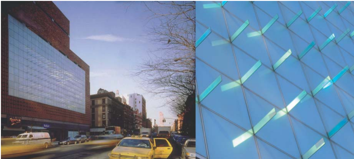
▲ Figure 7-2 Dichroic light field from James Carpenter Design Associates. To animate a blank, brick façade, a field of 216 dichroic fins was attached perpendicularly to a large plane of semi-reflective glass
