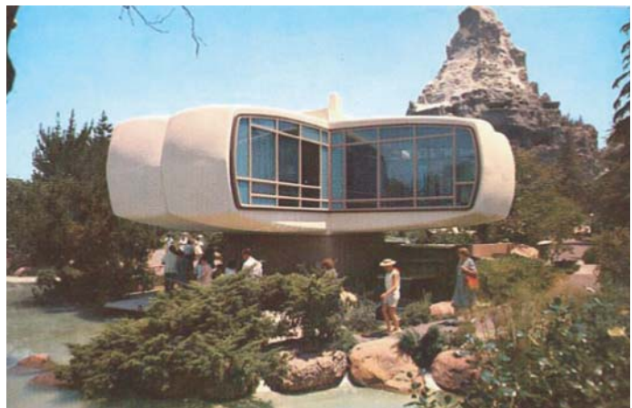
▲ Figure 8-1 Monsanto's 'House of the Future' opened at Disneyland in 1957. The house, and all its furnishings, were fabricated of plastic
