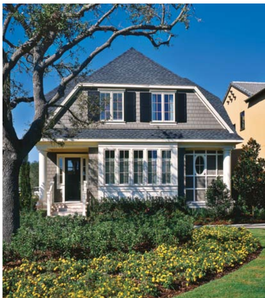
Our New Urban Challenge project, built at the height of the housing boom, challenged architects to do more with less in a production neighborhood setting. One of three homes built for the project, this Dutch Colonial-style home was designed by Bill Kreager for an empty-nester couple. Critical elements included a first-floor master bedroom, formal dining space (behind those front box windows), and a side porch.
