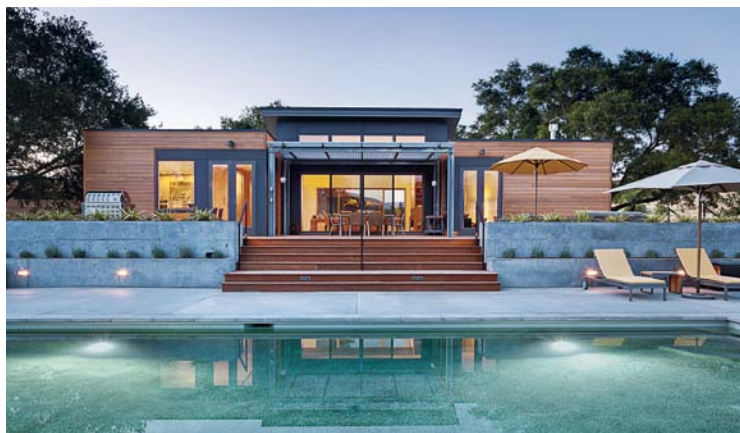
In Michelle Kaufman's Breezhouse, two factory-built modules are connected by a site-built breezeway. Glass wall panels open accordion-style to merge the central living area with a patio and the outdoors. Buyers may select among six siding styles. The home is now available from Blu Homes.
