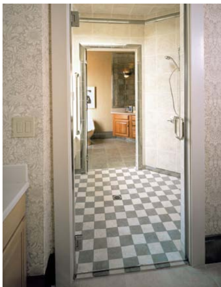
The LifeStages Home included a “roll-through” shower without a door threshold that worked well for people of all physical abilities. Once inside, detachable showerheads, coupled with overhead sprays and a bench for sitting or storage, made showering easy and enjoyable.
