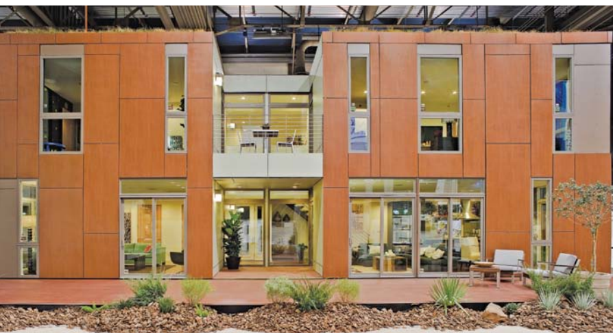
The Builder LivingHome , assembled in three and a half days on the floor of the 2009 International Builders Show, demonstrated the appeal of modular housing. Based on a design by KieranTimberlake, the home consisted of four modules joined by a breezeway. Smart panels that held the home's electrical and plumbing components could be snapped in place.
