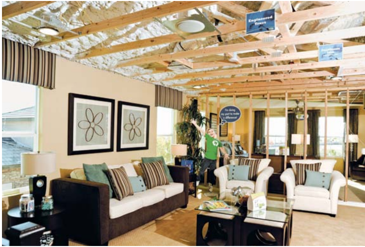
Deconstructed model homes by Meritage invite homebuyers to look behind the walls and learn from technology displays. During the downturn, progressive builders called attention to how they built homes, highlighting high-performance features such as heat-recovery ventilators, spray foam insulation, and post-tension slabs rarely found in less-efficient resale homes.
