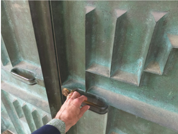
Eliel Saarinen, Cranbrook Art Museum, Bloomfield Hills, Michigan, 1942 The door handle is part of a solid bronze casting. It brings together the functional, aesthetic and tactile language of the building.
