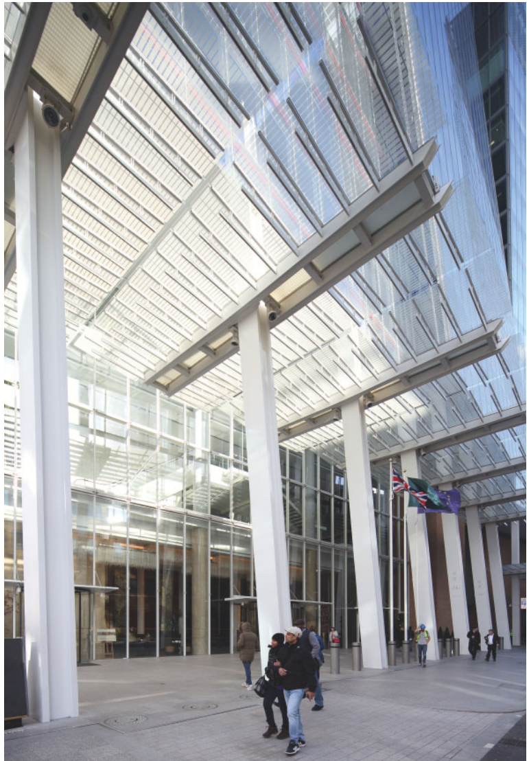
Renzo Piano, The Shard, London, 2013 The 'legs' of the Shard seem very thin in proportion to its bulk.
