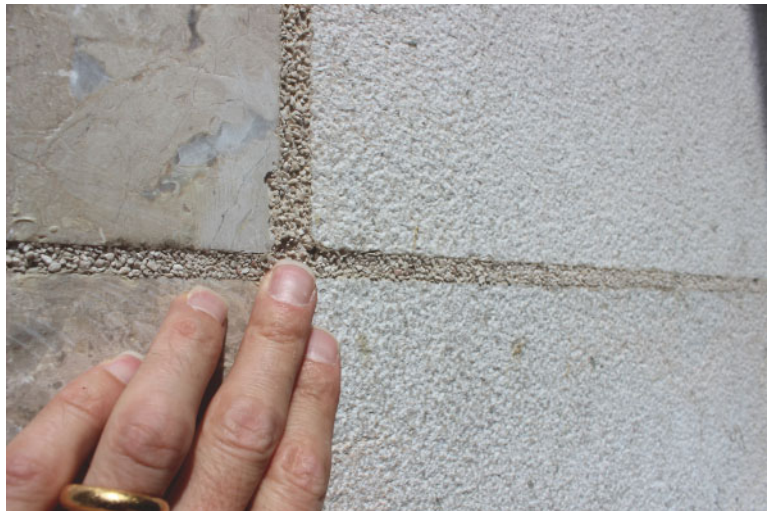
Allies and Morrison, Amiri Diwan Quarter, Doha, for Msheireb, 2014 Stone granules pressed into the silicone joints give the surface of a man-made chemical material, a natural and tactile feel.
