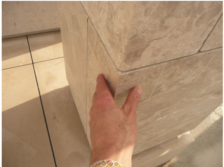
Allies and Morrison, Amiri Diwan Quarter, Doha, for Msheireb, 2014 The 150-millimetre (6-inch) stone return gives a sense of solidity throughout.
