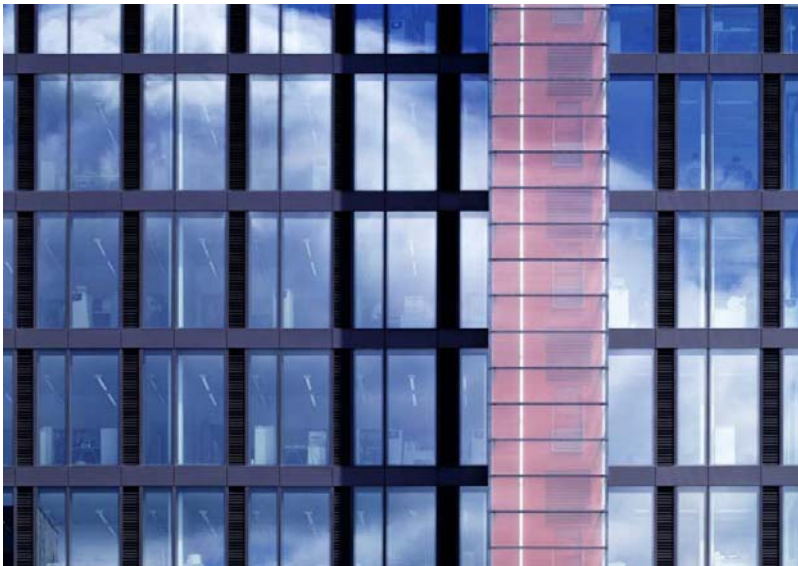
Figure 14 – Final hybrid façade with twin faces façade parts with integrated movable sunsreen and individual operable windows behind the fixed sunscreens
