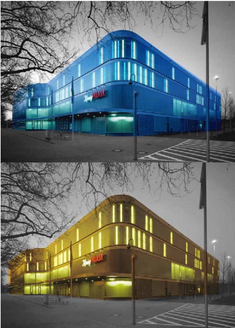
Figure 18 - 19 - Main façade of the ice stadium with the alternative illumination scenarios to generate branding for different uses – ice hockey games or concerts. The change of the colors of the lightning expresses the different uses: ice blue for hokey to amber for concerts.
