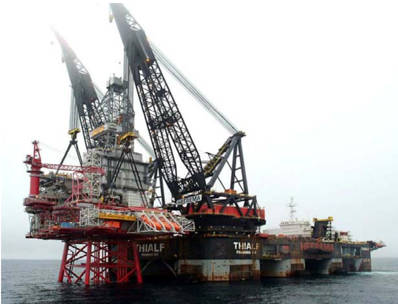
Fig. 6 Installation of prefabricated integral topside facilities.
