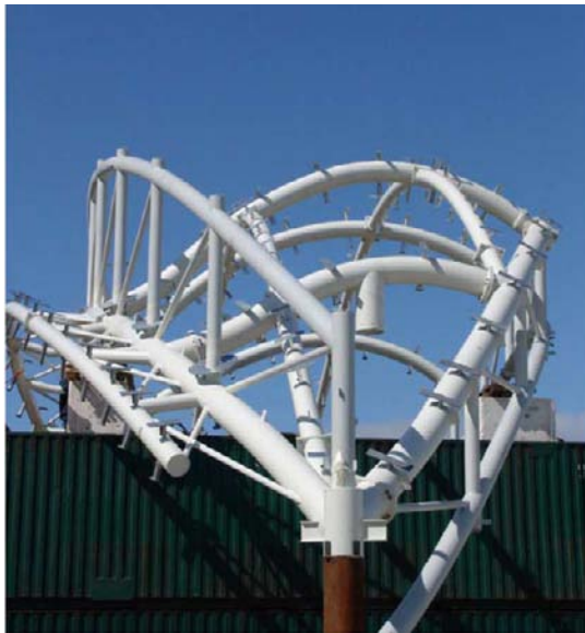
Fig. 39-40. The central body of the Great Hall (spanning ca. 30m)
