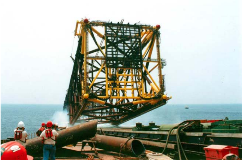
Fig. 15. Compliant tower just before leaving the barge.
