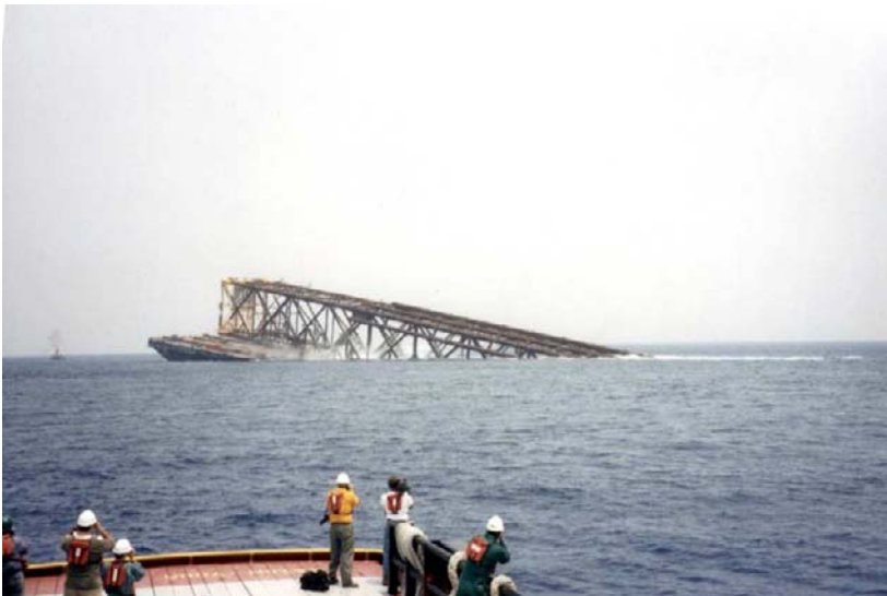
Fig. 14. Compliant tower sliding from the barge.
