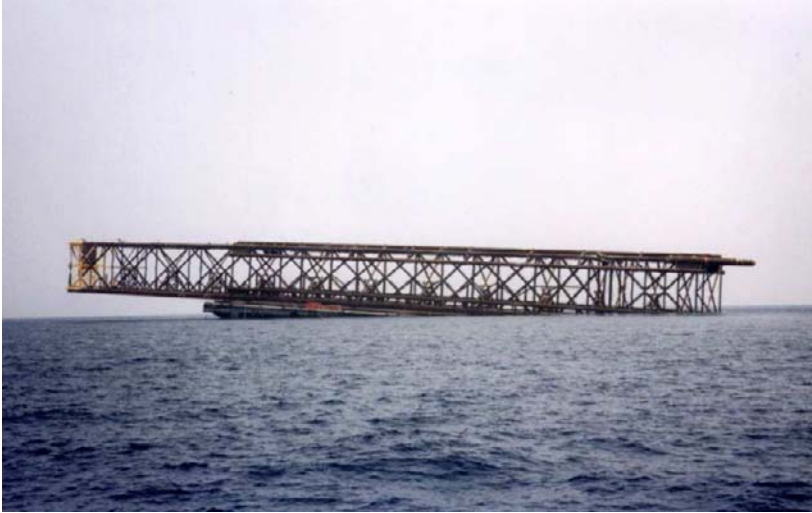
Fig. 13. Preparation for launching the compliant tower.
