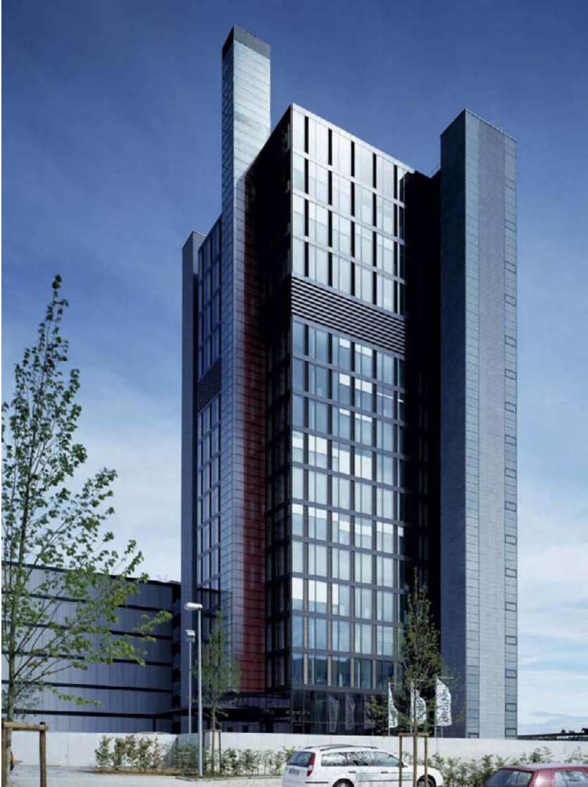
Figure 7 – Main entrance and solar chimney of the high-rise part of the building complex debitel
