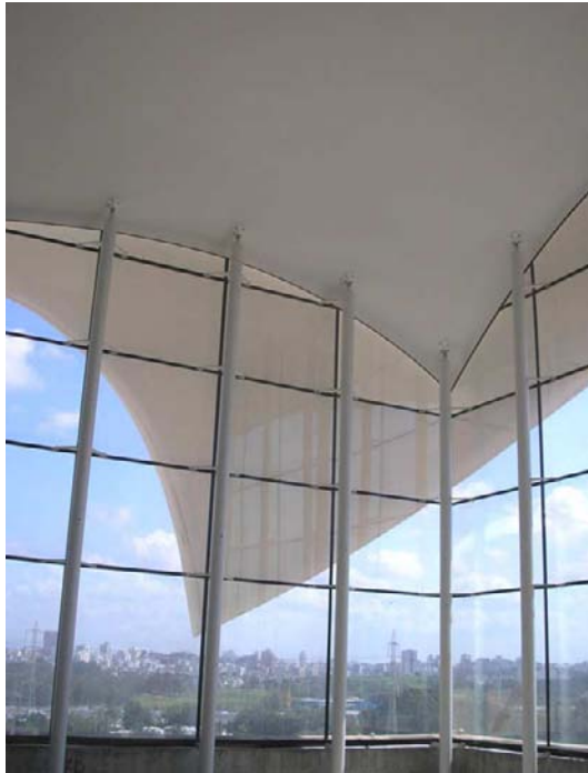
Fig. 56. The Great Hall Interior view
