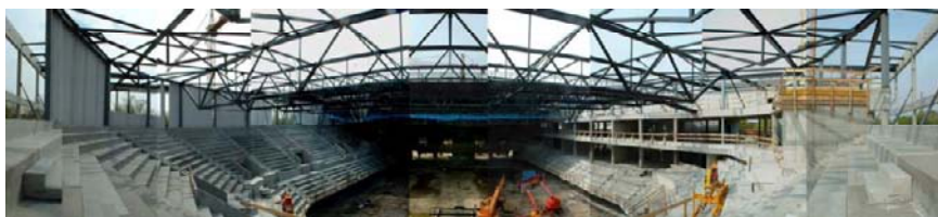
Figure 16 - Interior during construction process
