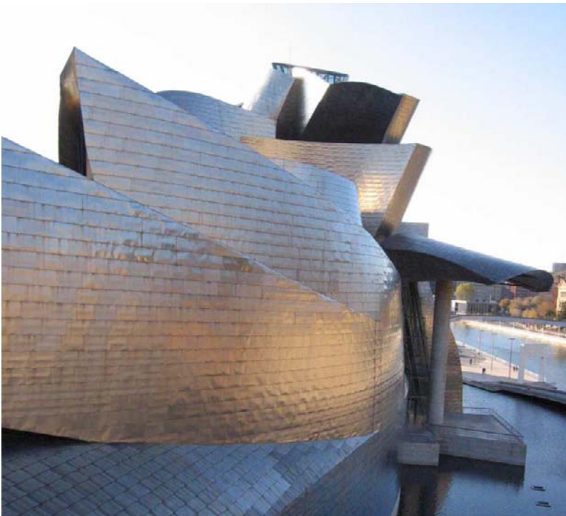
Figure 20 - Guggenheim Museum by Frank O. Gehry in Bilbao
