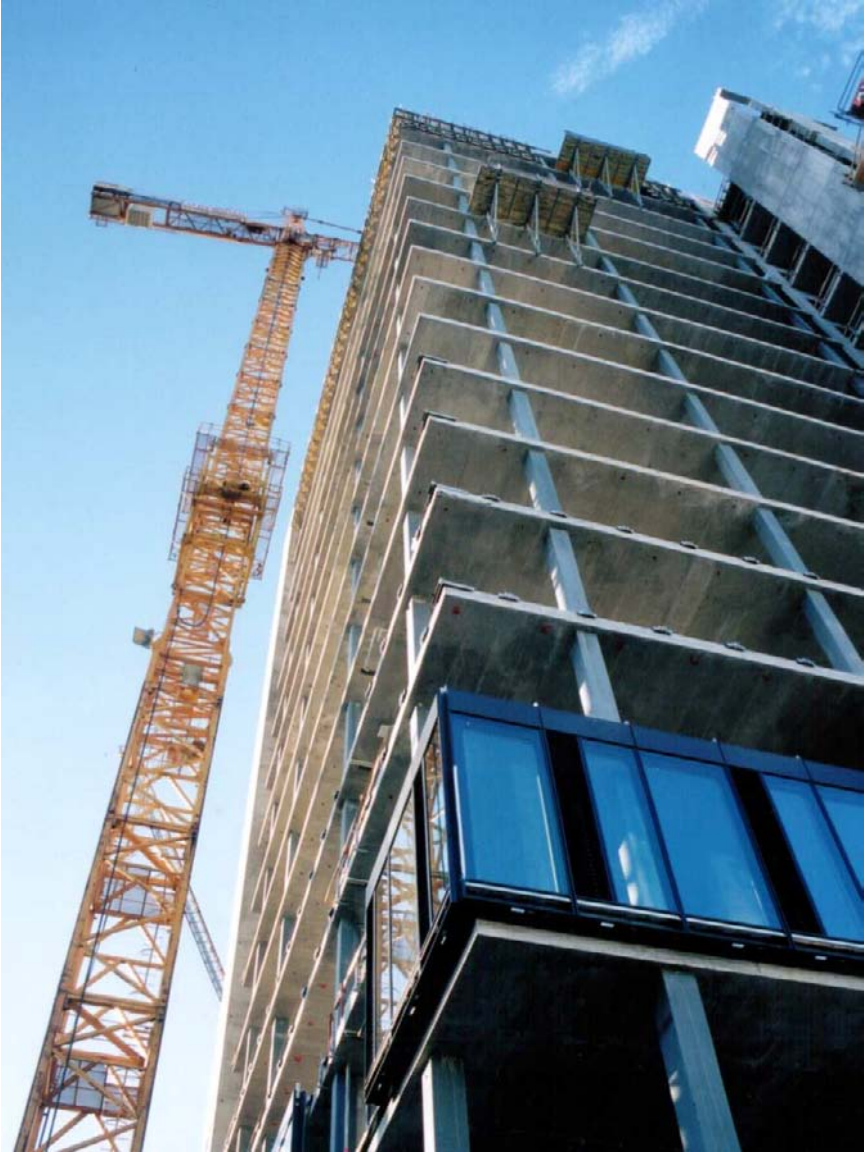
Figure 15 – Construction side of the hybrid façade
