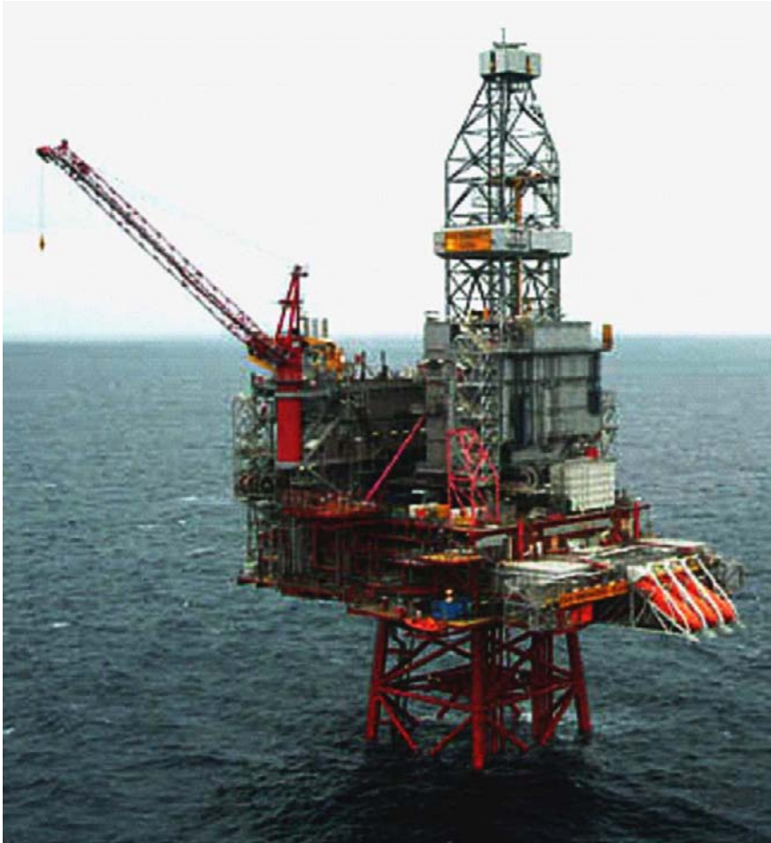
Fig. 1. Production facilities on a bottom founded fixed platform.
