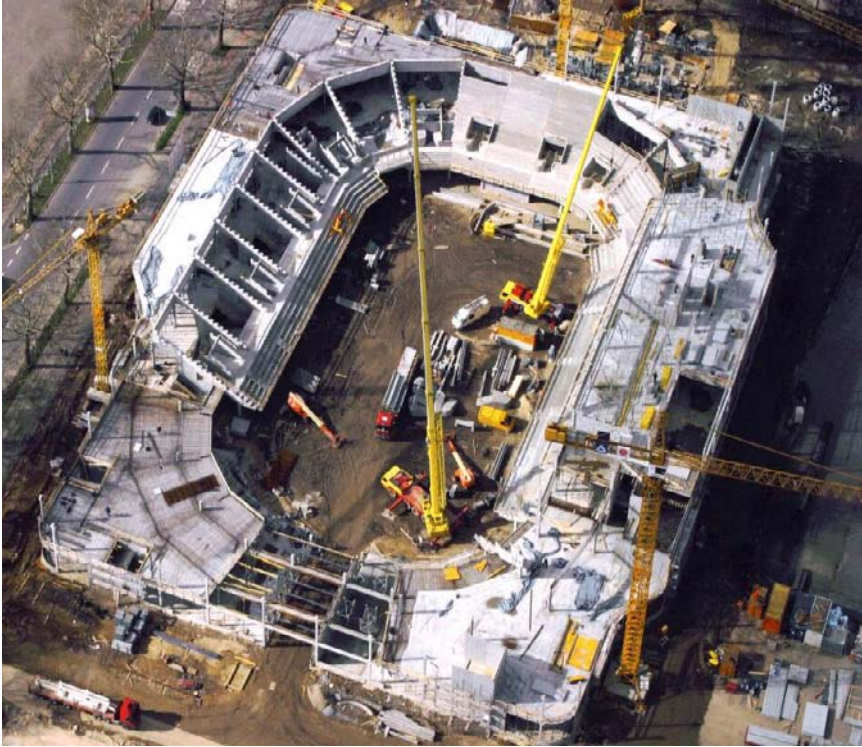
Figure 17 Bird's eye view of the ice stadium / Krefeld during building process.
