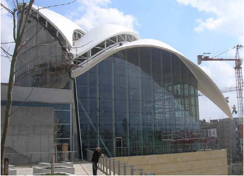
Fig. 55. Finishing of the top layer of the roof by "airborne builders"
