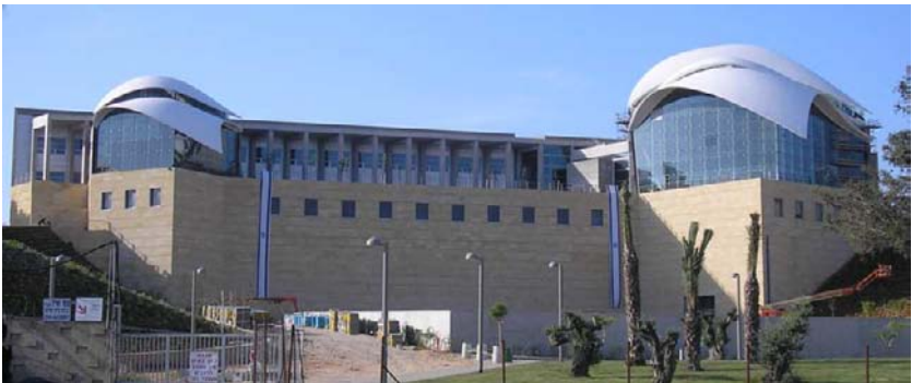
Fig. 52. View of the building site in April 2006.
