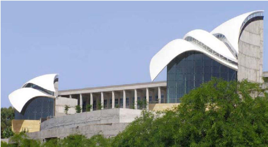
Fig. 54. Overview of the building site just after completion of the roofs by Octatube.
