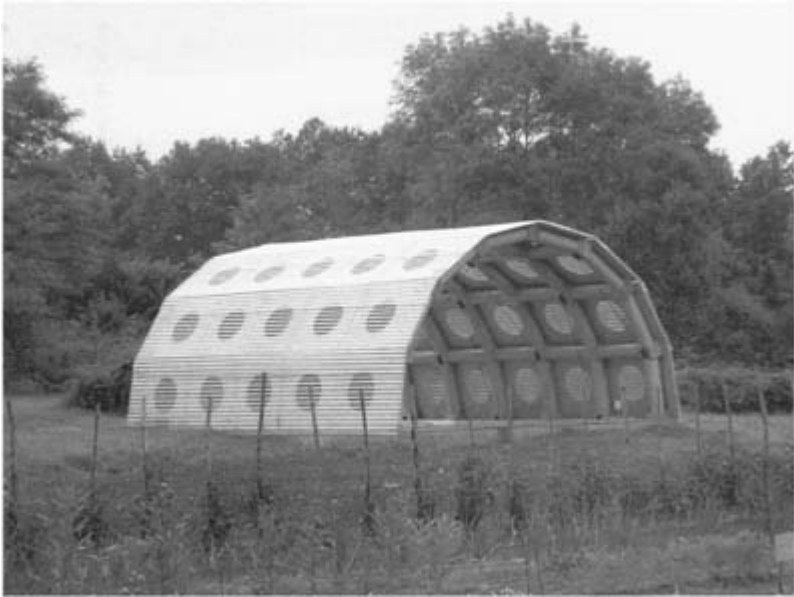
11.4 Paper arch designed by Shigeru Ban and built in 2001 at the Vitra design workshops run at Domain de Boisbuchet, Lessac, France
