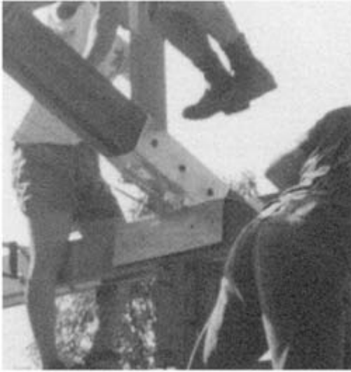
8.14 Truss-beam-column connectors
