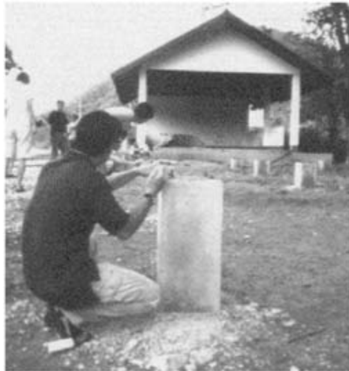
8.6a Construction of footings
