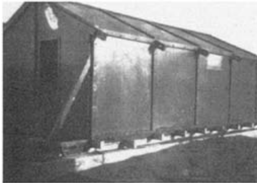
7.6 The completed structure with end braces
