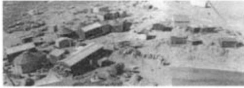
7.3 Atlas Coves Station, Heard Island, 1951. A 14-sided Alaskan hut is seen on the left with an ANARE Mark 1 behind it and a Borden building behind the Mark 1
