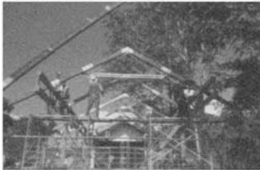
8.17 Fitting truss onto vierendeel beam
