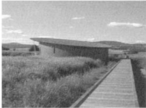
10.4 The permanent replacement building
