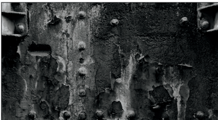
Here, they're darkened to almost match the surrounding rust
