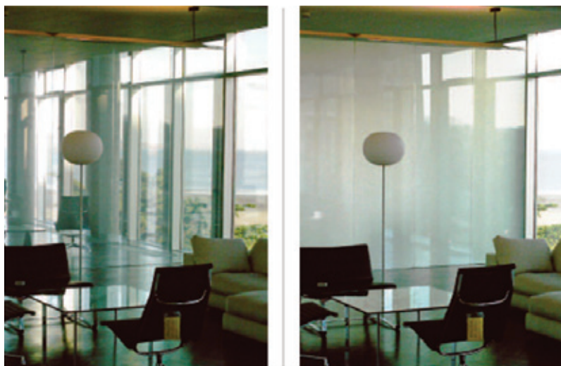
FIG 1.5: Now you see it, now you don't: smart glass can be configured to become opaque automatically ( http://bkaprt.com/rwd/7/ ).
