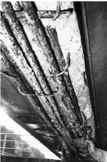
*Figure 2.12* When the concrete cover in the lower parts of the deck beams had cracked or spalled off at a very early stage, the steel bars were more uniformly corroded, while the protruding beam stirrups always showed a more pitting-type of corrosion (source: Gjrv (1968)).
