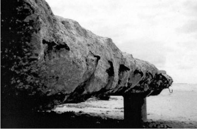
*Figure 2.30* Remaining part of the deck from the concrete pier built on the Yocatán Coast in the 1960s (source: Courtesy of Rambøll Consulting Engineers).
