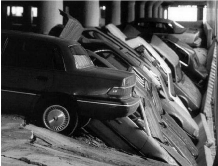
Figure 2.62 The consequences of corrosion in garages exposed to de-icing salt contamination have occasionally been quite severe (source: Courtesy of Sten H. Vælitlalo).
