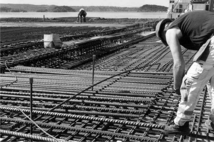
Figure 11.5 The concrete deck had very congested reinforcement.
