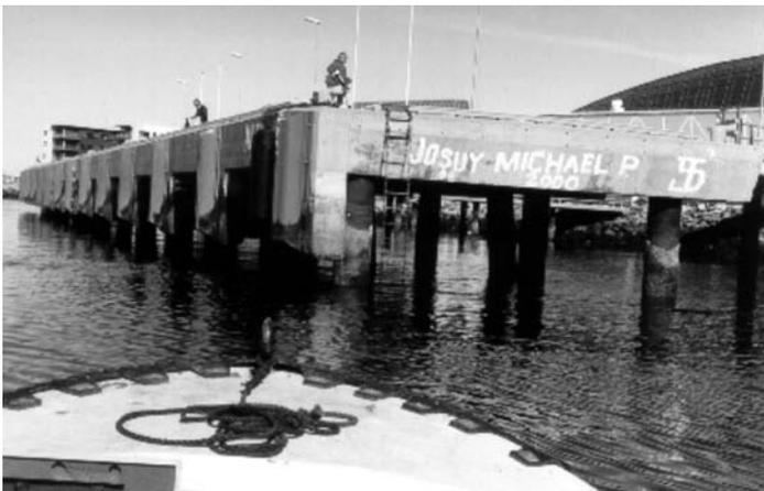
Figure 2.20 'Turistskipskaia' (1993) in Trondheim Harbour with steel corrosion in most of the deck beams after eight years of exposure (source: Gjrv (2002)).
