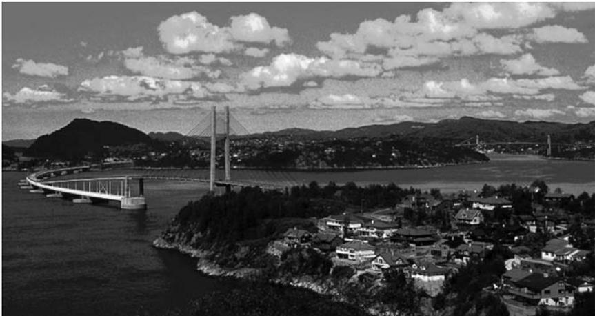
*Figure 1.6* The Nordhordlands Bridge (1994) is a combined floating and cable-stayed bridge with a total length of 1610 m (source: Courtesy of Johan Brun).
