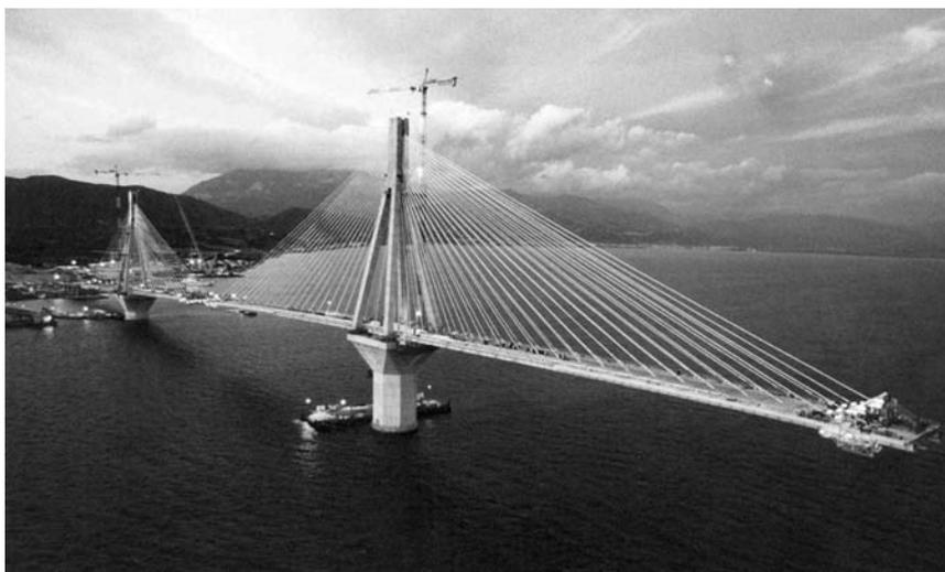
Figure 1.14 The Rion–Antirion Bridge (2001), to which a concrete with an extremely high resistance to chloride penetration was applied (source: Courtesy of Gefyra S.A.).
