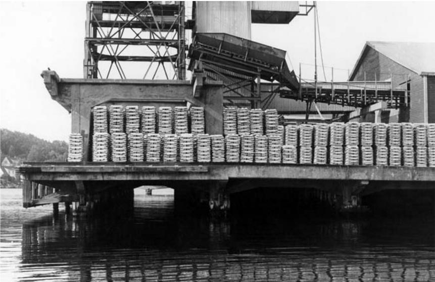
*Figure 2.6* A 50-year-old industrial harbour structure (1913) with storage of raw aluminium bars representing an evenly distributed deck load of approximately six times that of the original design load (source: Gjørnv (1968)).
