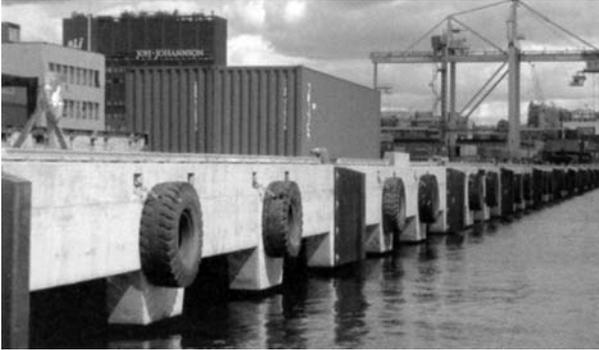
Figure 2.27 During construction of ‘Nye Filipstadkaia’ (2002) in Oslo Harbour, deep chloride penetration in several of the deck beams took place due to heavy winds and high tides (source: Courtesy of Oslo Harbour KF).
