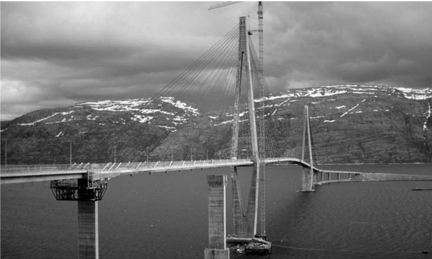
*Figure 2.46* The Helgeland Bridge (1991) is a 1065 m-long cable-stayed bridge with the largest span of 425 m (source: Courtesy of Hallgeir Skog).
