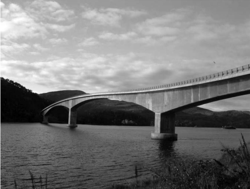
Figure 2.49 The Aursundet Bridge (1995) is a cantilever bridge with a total length of 486 m.
