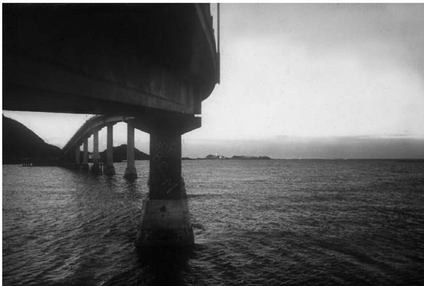
*Figure 2.35* Ullasundet Bridge (1970) was demolished after 25 years of service due to heavy corrosion of embedded steel (source: Courtesy of Jørn A. Hasselø).
