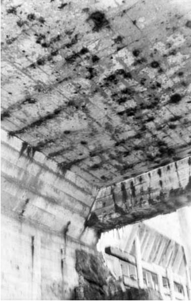
*Figure 2.11* The rear parts of the concrete deck adjacent to the seawall were more vulnerable to steel corrosion than the rest of the deck (source: Gjrv (1968)).
