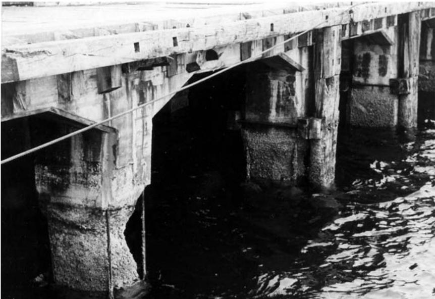
*Figure 2.9* Uneven deterioration in the tidal zone due to the high variability of concrete quality from one pillar to another (source: Gjørøv (1968)).
