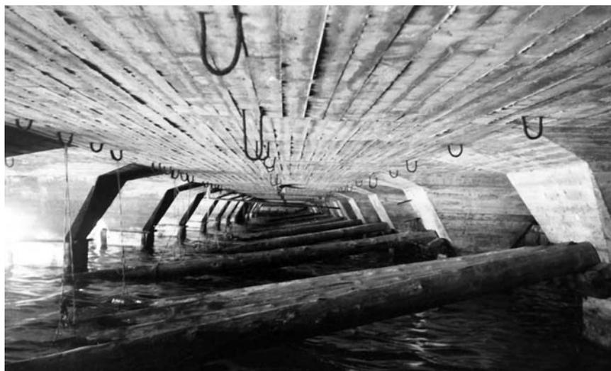
Figure 2.13 Harbour structures with a concrete deck of the flat type showed a much better performance than structures with a beam and slab type of deck (source: Gjørø (1968)).
