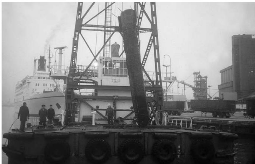
*Figure 2.18* Four of the tremie-cast concrete pillars from the concrete jetty in Oslo Harbour (1922) were pulled up on shore for a more detailed investigation.
