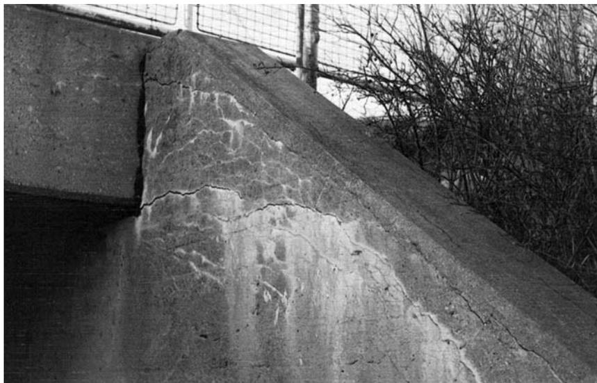
*Figure 4.2* Typical damage due to alkali-aggregate reaction in a retaining concrete wall of a bridge.
