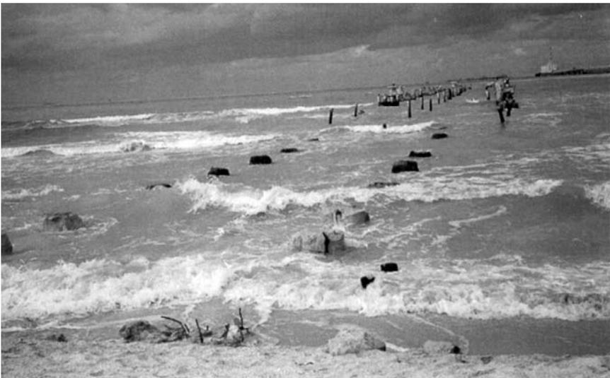
Figure 2.29 Remaining parts of a concrete pier built in a conventional way on the Yucatán Coast in Mexico in the 1960s (source: Courtesy of Rambøll Consulting Engineers).
