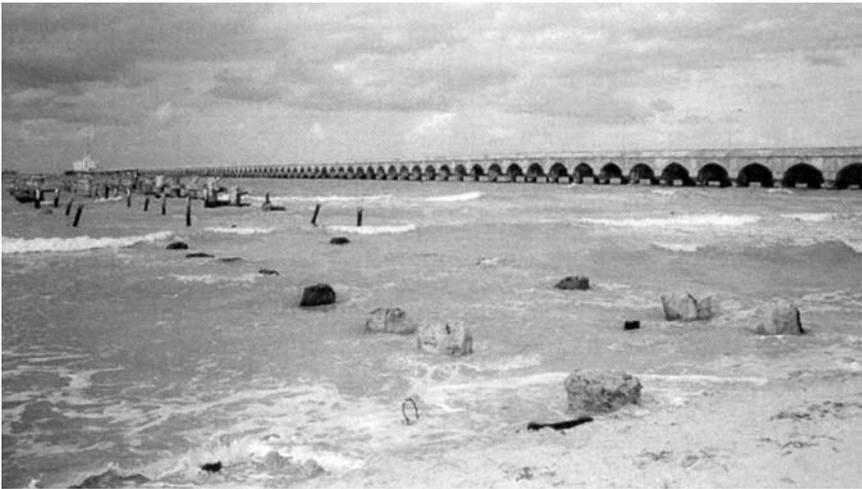
*Figure 2.31* Different durability and long-term performance of the two concrete piers on the Yocatán Coast built with black steel in the 1960s (front) and with stainless steel during 1937–1941, respectively (source: Courtesy of Rambøll Consulting Engineers).
