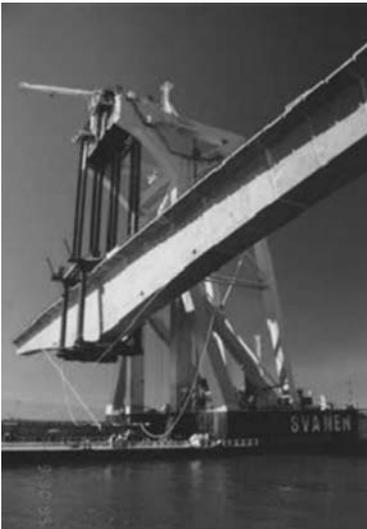
Figure 7.7 Precast cantilever girder for the Northumberland Strait Bridge.
