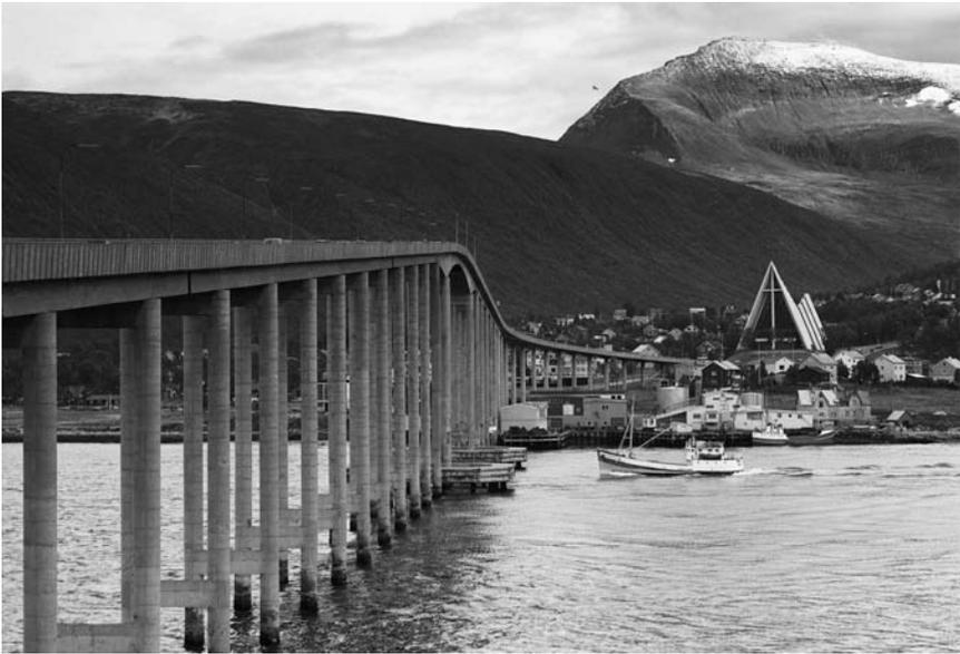
Figure 1.4 The Tromsø Bridge (1960) is a cantilever bridge with a total length of 1016 m (source: Courtesy of Johan Brun).
