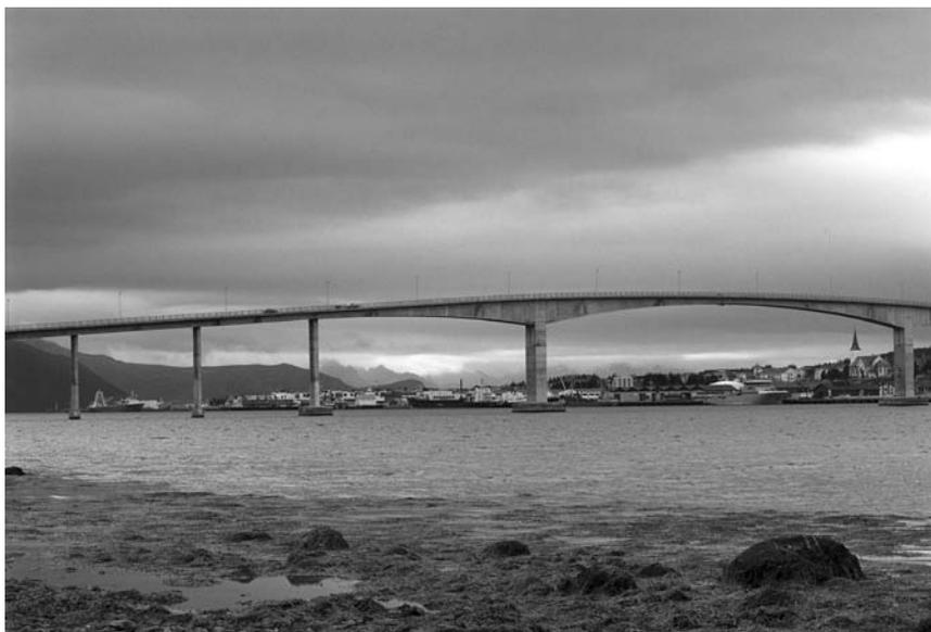
*Figure 2.1* The Sortland Bridge (1975) is a 948 m-long cantilever bridge in the northern part of Norway (source: Courtesy of Johan Brun).
