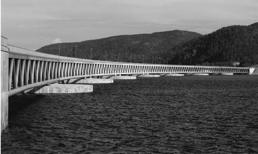
*Figure 1.5* The Bergsøysund Bridge (1992) is a floating bridge with a total length of 931 m (source: Courtesy of Johan Brun).
