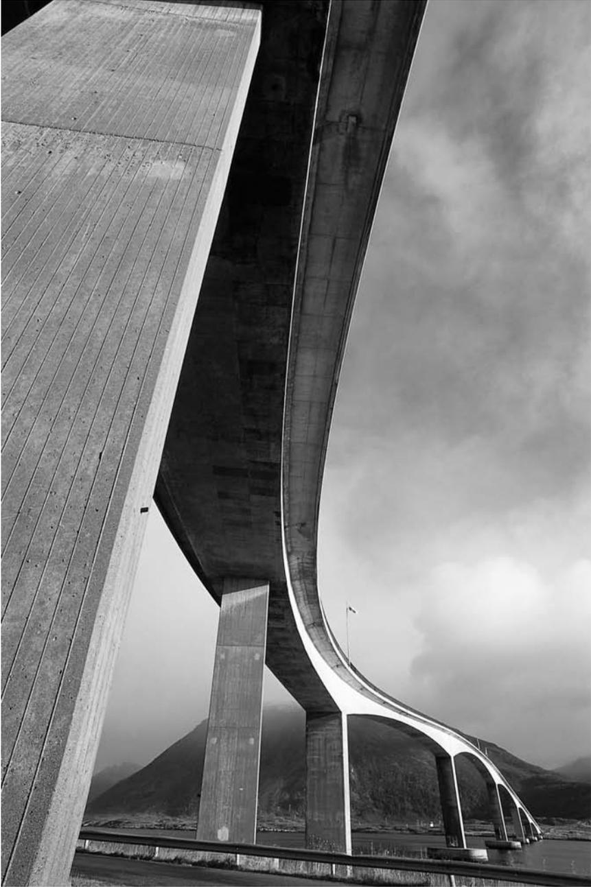
*Figure 2.36* Gimsøystraumen Bridge (1981) which was the most common type of Norwegian concrete coastal bridge from the 1970s and 1980s (source: Courtesy of Johan Brun).
