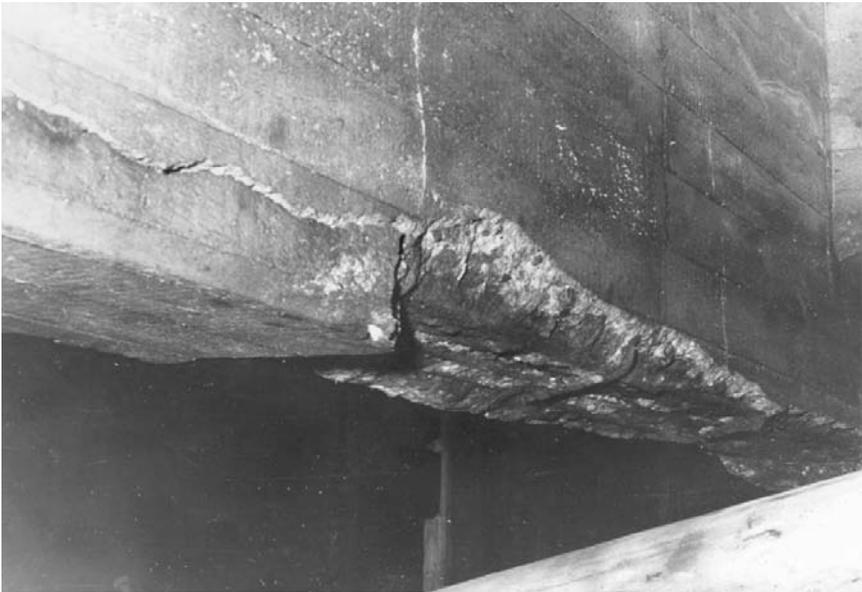
*Figure 2.10* The lower parts of the deck beams were more vulnerable to steel corrosion than the deck slabs in between (source: Gjørv (1968)).
