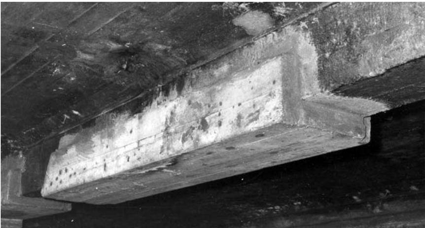
Figure 2.14 Typical patch repair of a corroded deck beam (source: Gjørnv (1968)).
