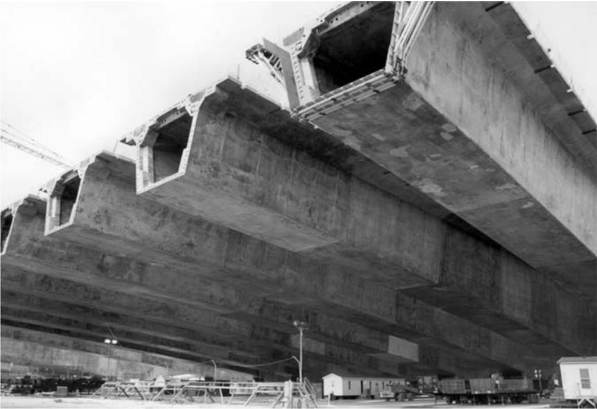
*Figure 7.8* Precast cantilever girders for the Northumberland Strait Bridge.
