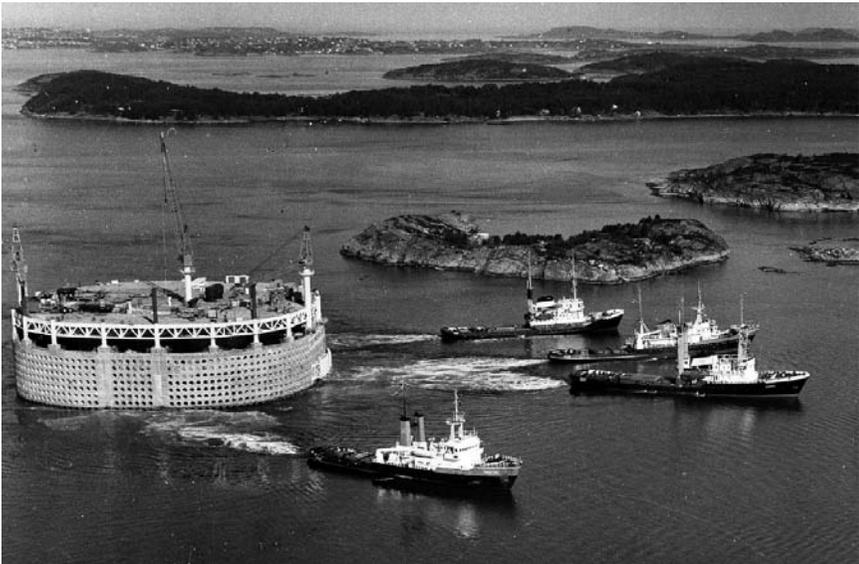
*Figure 1.8* The first offshore concrete platform, the Ekofisk Tank, on its way out of Stavanger in 1973 (source: Courtesy of Norwegian Contractors).
