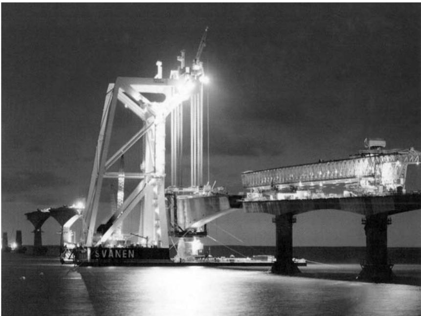
*Figure 7.9* Installation of cantilever girders for the Northumberland Strait Bridge (source: Malhotra (1996)).
