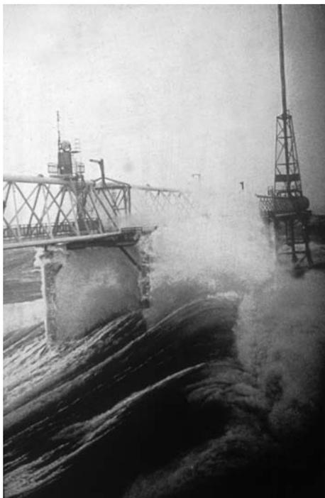
*Figure 2.52* All the concrete platforms in the North Sea are exposed to heavy wave loading.
