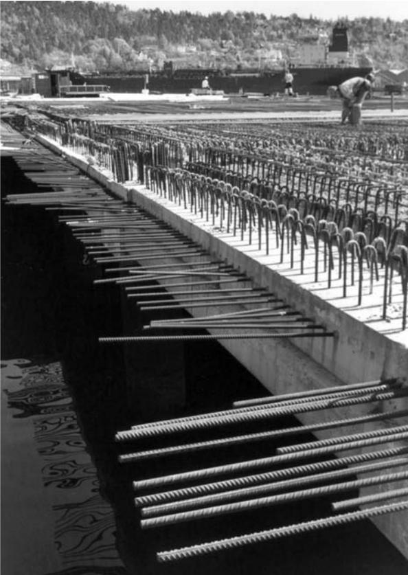
Figure 11.4 Protruding bars in the joints of the concrete deck.
