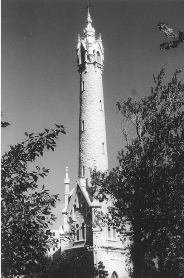
The Gothic Old North Point Water Tower, built 1871–73 in Milwaukee, stored water for that city's system. Such towers were a prominent civic feature of cities ranging in size from Chicago to Fresno, California. Photograph by the author.
