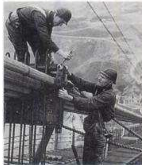
The main cables used in suspension bridges should not be intertwined, but parallel, so that they can move slightly alongside each other. This excludes the occurrence of bending stiffness.
