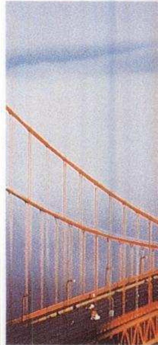
The main cables used in suspension bridges should not be intertwined, but parallel, so that they can move slightly alongside each other. This excludes the occurrence of bending stiffness.
