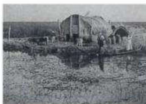
Reed without a trace of matrix material, but bundled and shaped in the most obvious way, is used to build ultra light swamp huts.
