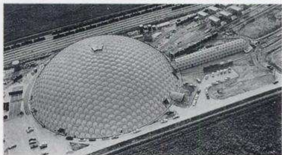
Building a geodesic dome is a repeating of modular elements.
