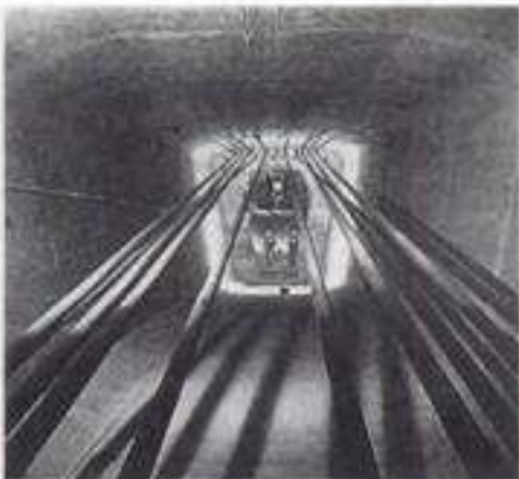
This kind of anchor at the end of a steel cable is difficult to translate into a solution for carbon cable anchoring.
