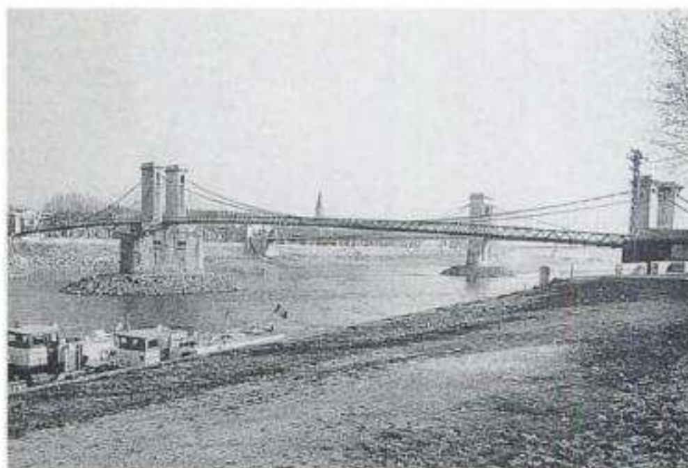
In several of these (bicycle chain) bridges in France the steel deck was replaced by an aluminium one to increase the payload.
