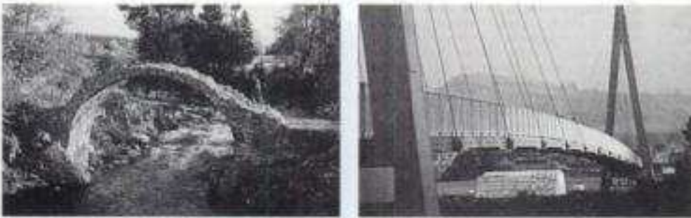
This old Celtic bridge in Scotland demonstrates the carrying capacity of a worn down arch. Scotland also has a full composite bridge.
