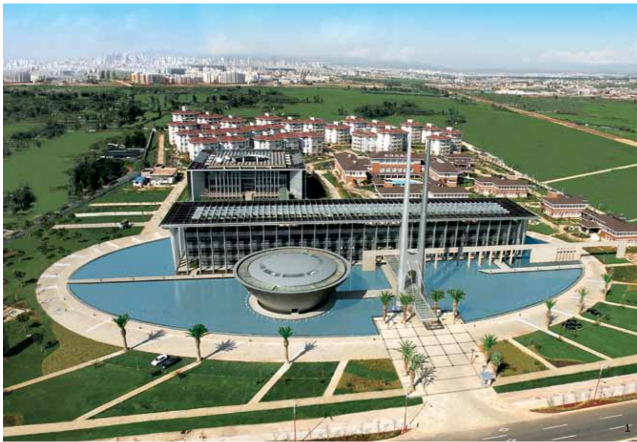
1. Bird-eye view of the whole region 2. The second floor plan 3. "H" shape structure at the entrance rising from the water
