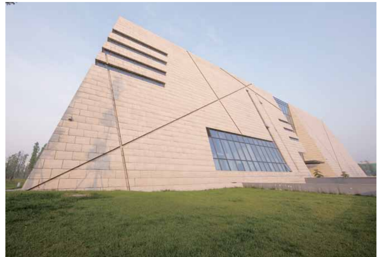
Close view of the museum, with dry-hanging travertine on the wall
