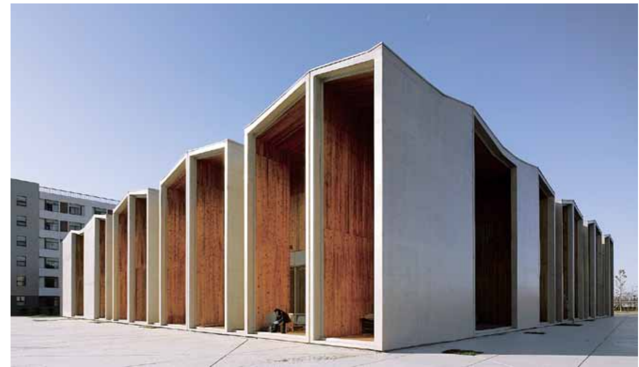
Exterior of the building
