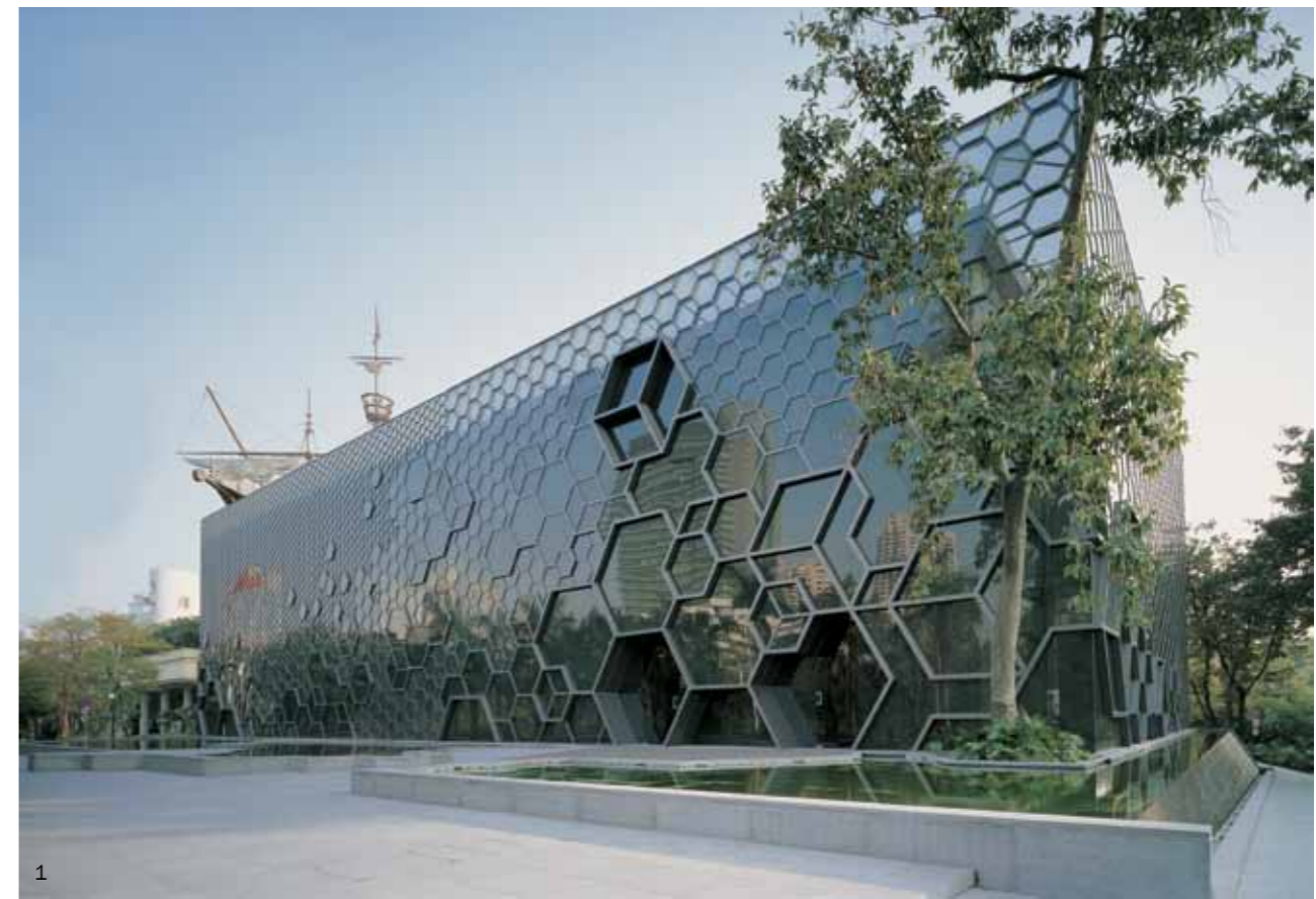
1. Full view of the building, and the exterior elevation being like "honeycomb" 2. Plan
