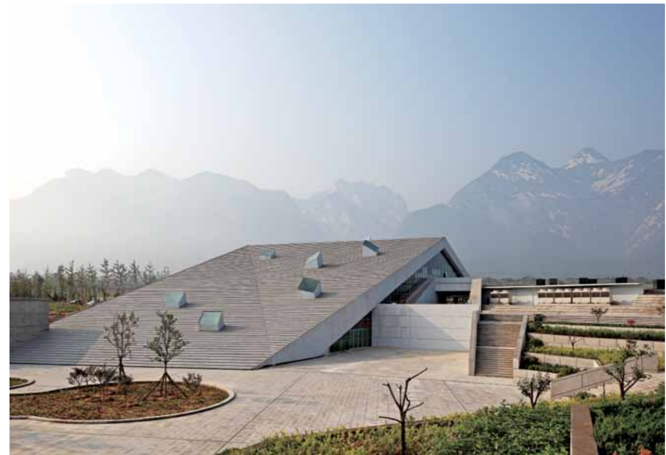
The sunken plaza and the step greening
