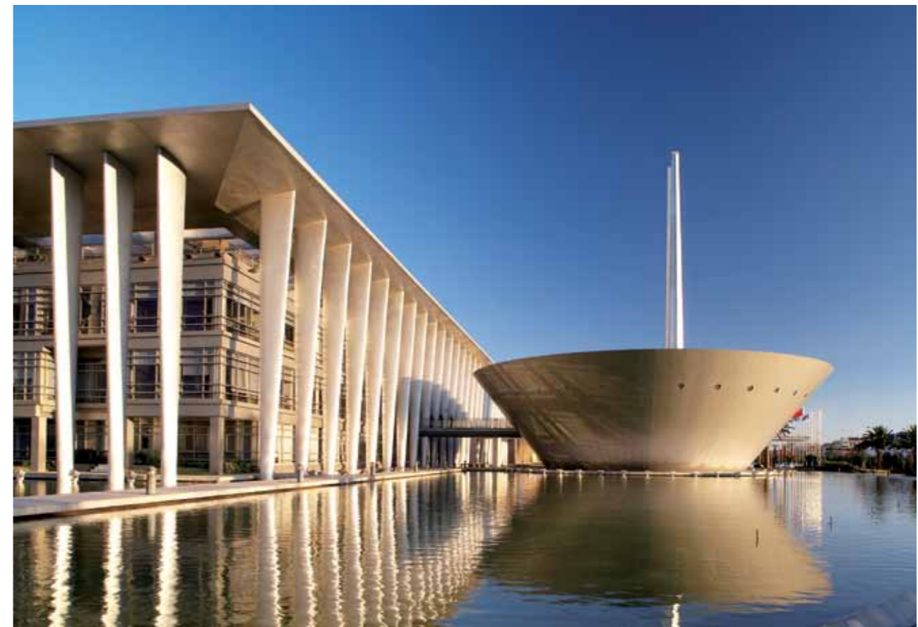
The appearance of the meeting area above the water
