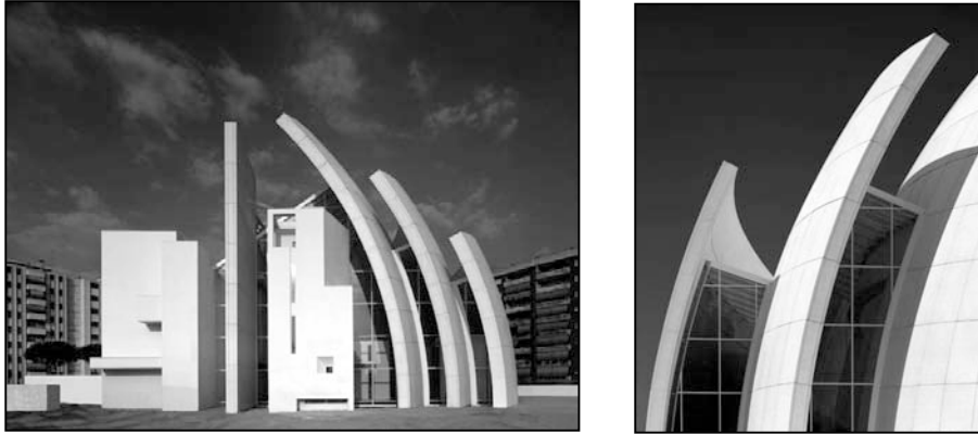
Figure 7: Façade of Ruby Jubilee Church, Rome where self cleansing concrete panels have been used.
