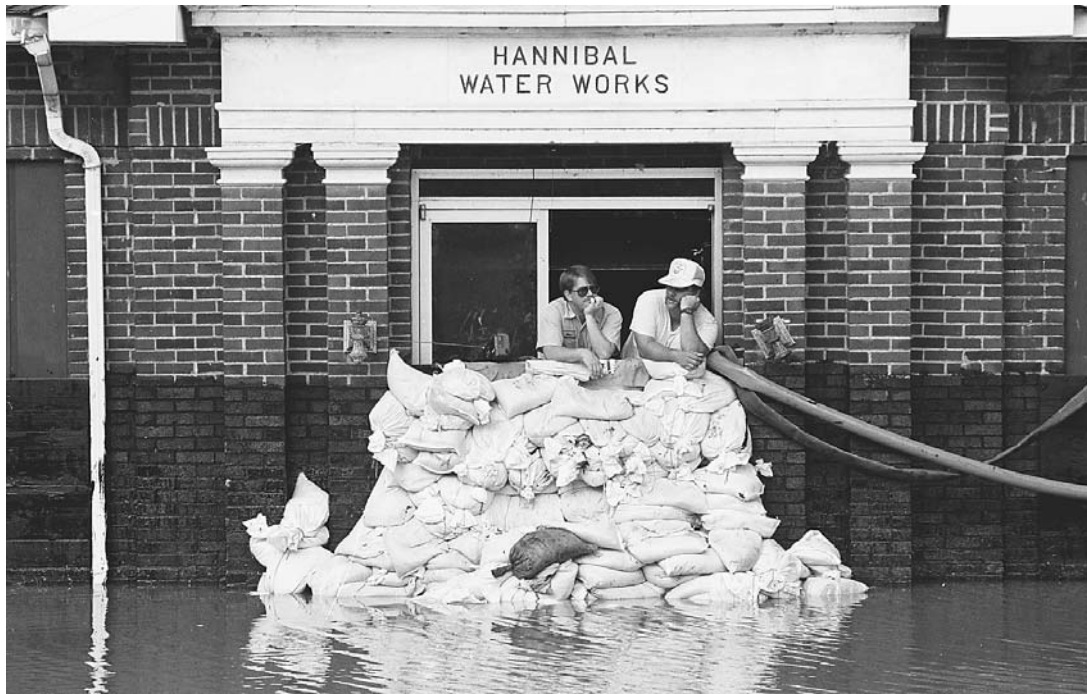
THE FLOODWATERS OF THE MISSISSIPPI RISE TO 4 FT. (1.2 M), SURROUNDING THE PUMPING STATION IN HANNIBAL, MISSOURI. APART FROM NATURAL CAUSES, FLOODS CAN RESULT FROM INCONSISTENT FLOOD MANAGEMENT, POOR CIVIL ENGINEERING DESIGN, AND UNWISE AGRICULTURAL PRACTICES. (AP/Wide World Photos. Reproduced by permission.)
