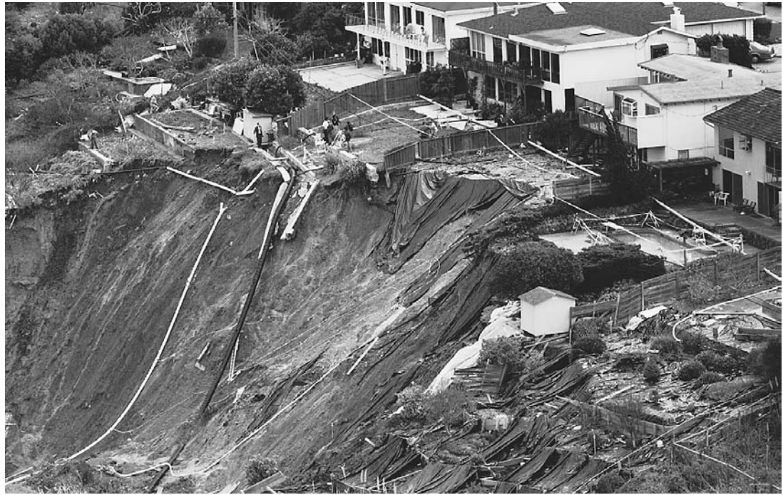
A MUDFLOW CAUSED BY HEAVY WINTER RAINS BRINGS DOWN THE HILLSIDE UNDER HOMES IN MILLBRAE, CALIFORNIA. (AP/Wide World Photos. Reproduced by permission.)
