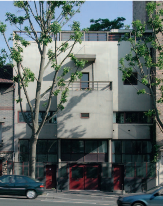
Figure 4.22: A building that complies with the principles for quick, accurate, and confident perception. Maison Planeix, Paris , by Le Corbusier, 1924–28. (Source: Gans, D., The Le Corbusier Guide: Revised edition , Princeton Architectural Press, 2000) (courtesy of Simon Glynn www.galinsky.com )
