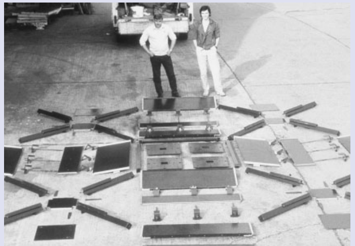
A set of the steel and plywood components used in the elemental formwork system for the Lloyd's floors.
