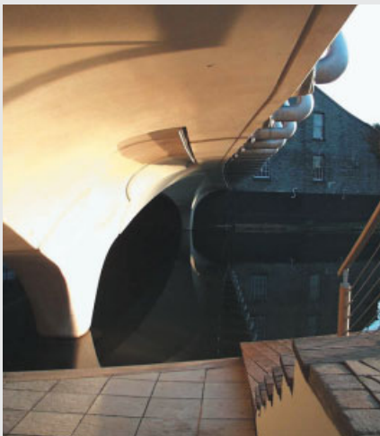
Detail of Ballingdon Bridge from the Sudbury bank.
