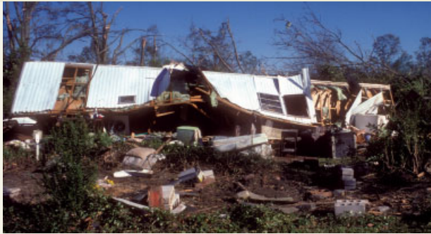
A mobile home following the attentions of a tornado in Alabama, us. The loss of life and property from the use of unsuitable and unsustainable timber structures is endemic. The economic calculations involved in making houses in the cheapest and fastest manner, using the minimum of labour and materials, are formidable. It is difficult to redirect this economic leviathan towards another way to produce human habitation.
