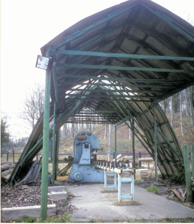
The simple structure shielding the circular saw at Hooke Park. Designed by students from the furniture school, it uses the material agenda of green round wood with intelligent simple joints to make a small, exemplary, useful building.
