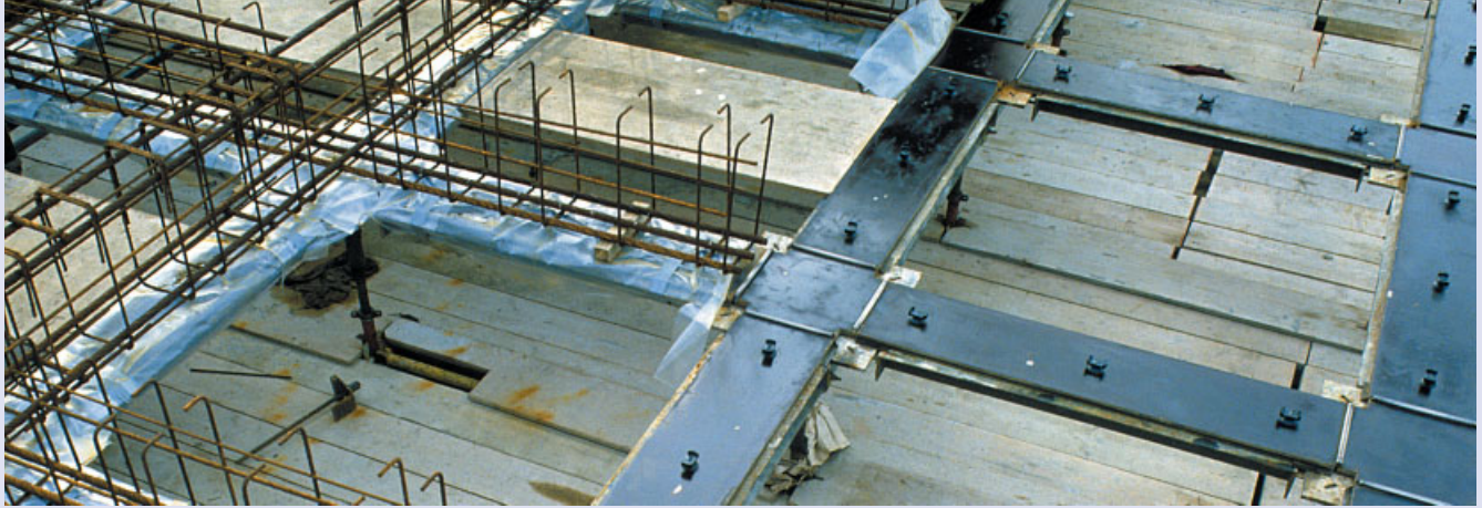
A section of assembled soffit forms showing the reinforcement support cradles for the Lloyd's floors. The raised strips at the intersections are the steel channels which contain the gaskets for the node/beam joints.
