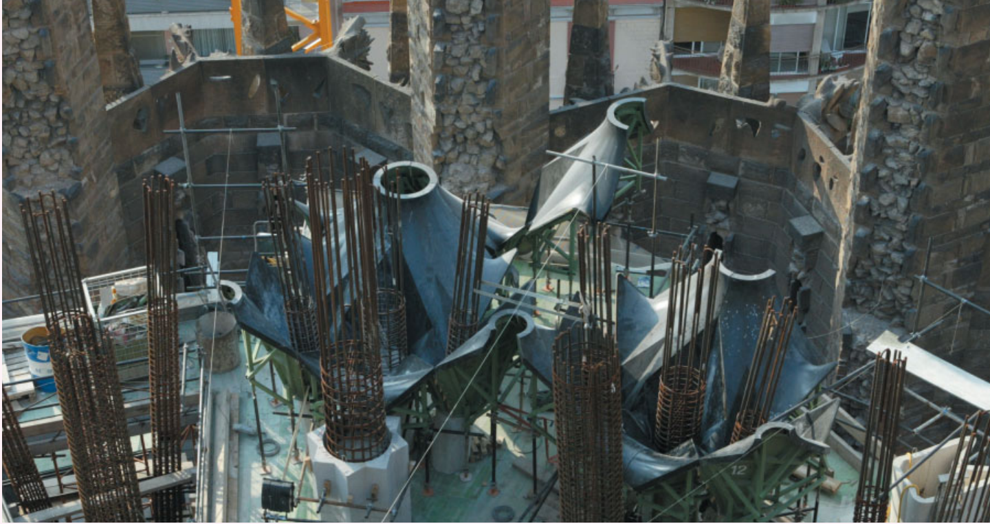
Positioning the fibreglass moulds above the ambulatory around the apse.
