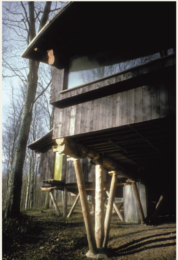
The Cullinan-designed accommodation block at Hooke Park. Adjacent are the footings for a fourth building that will be used to erect the first of the AA-commissioned structures.
