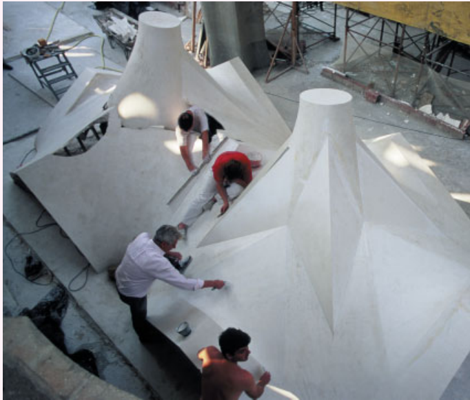
To make the mould-masters for the full-size components, Gaudí's process is simply scaled up using the same process that he used for his 1:25 and 1:10 scaled prototypes, and uses the same materials.
