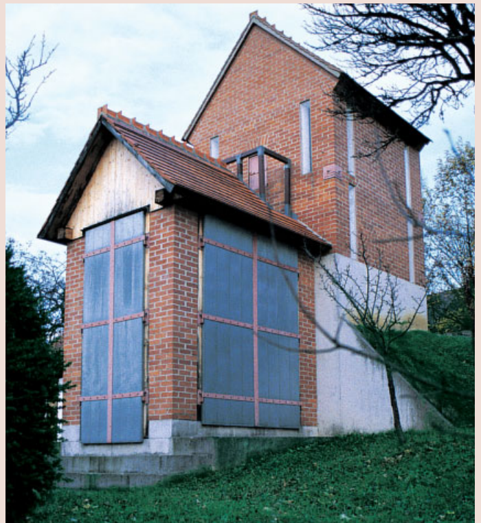
Small tower, Burgenland.
