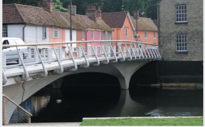
Ballingdon Bridge from the Sudbury bank.
