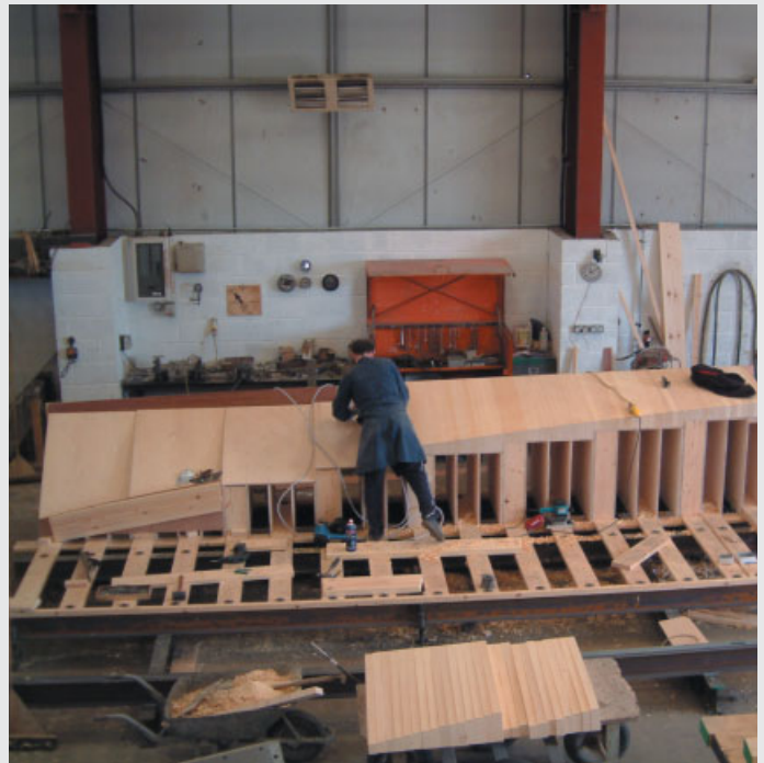
One of the precast-concrete models of Ballingdon Bridge under construction at Buchan's works in the West Midlands.
