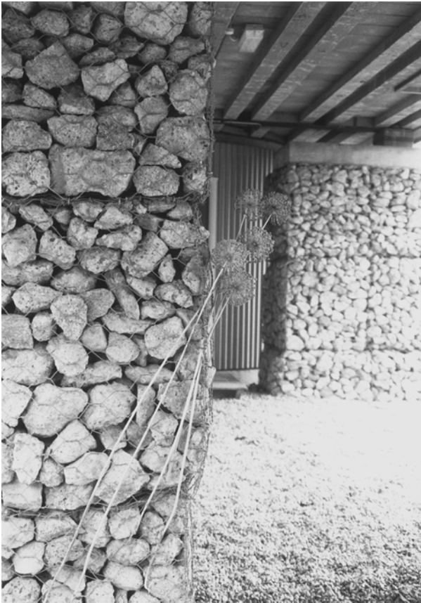
8.1 • Sarah Wigglesworth and Jeremy Till, 9/10 Stock Orchard Street , London, gabions containing recycled concrete
