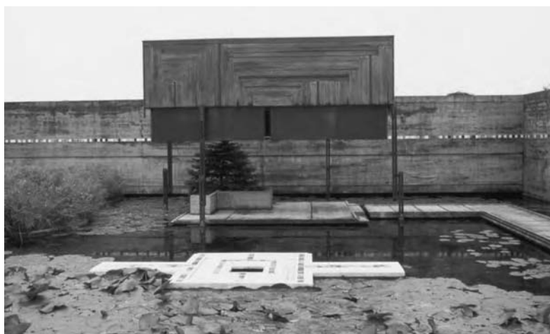
3.10 Carlo Scarpa, the Brion Cemetery, Italy, 1967-78. View of the pavilion and "propylaea".
