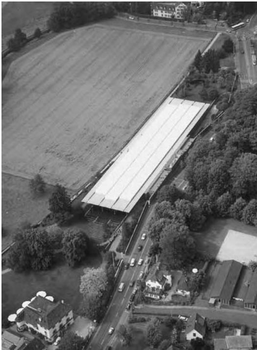
6.8 Renzo Piano, Foundation Beyeler, Riehn, 1994-97. Aerial view.
