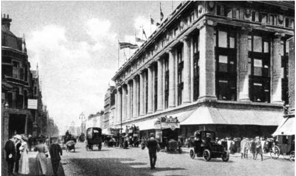
Selfridges department store, Oxford Street, London, 1909. Department store architects deployed varied, but predominantly classical, styles to represent the commercial ambitions of prestigious stores located on main city thoroughfares.
