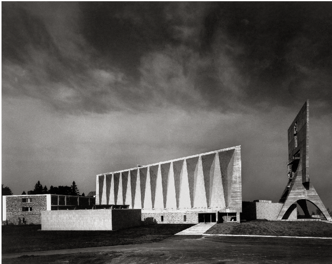
40. Saint John's Abbey Church, showing folded concrete wall
