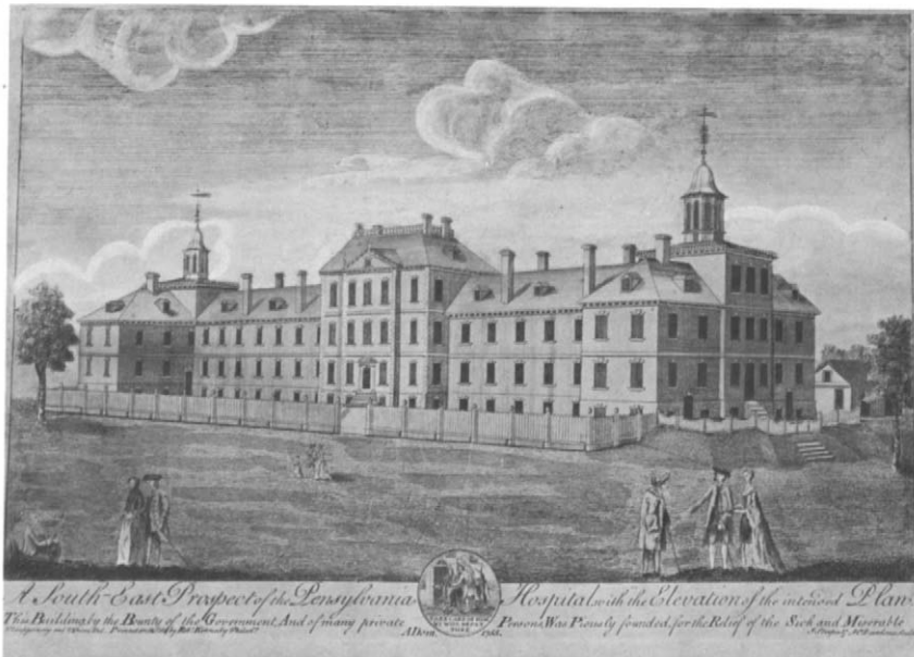
INSCRIBED: (at the bottom) A South-East Prospect of the Pennsylvania Hospital, with the Elevation of the intended Plan./ This Building, by the Bounty of the Government, And of many private Persons, Was Piously founded, for the Relief of the Sick and Miserable; (at lower left) Montgomery and Winter Del. Printed and Sold by Robt Kennedy Philada; (at lower center) A Dom, 1755; (at lower right) J. Steeper & H Dawkins Sculp; (in a small rondel inset [seal of the hospital] at lower center) TAKE CARE OF HIM/ & I WILL REPAY/ THEE.
